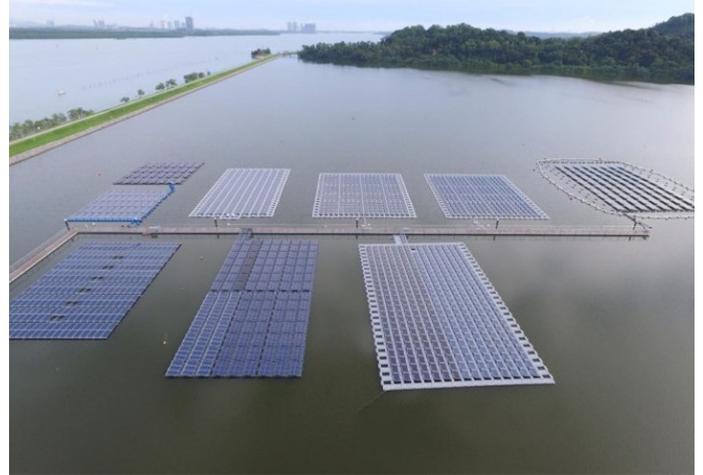
The site has numerous sensors and two meteorological stations, with more than 500 parameters monitored in real time across the complete installation. After the first test period, all systems achieved a performance ratio (PR) within the range of 78% to 94%, with the majority reaching PRs values of well above 80% - something not easy to achieve in the hot and humid climate of Singapore.
