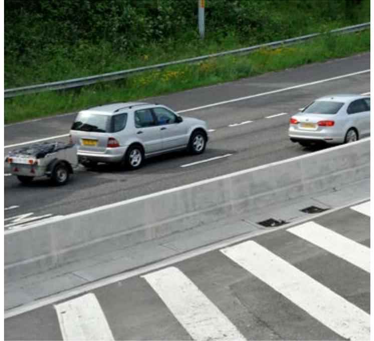
Sika concrete admixtures are playing an important role in the upgrading of central crash barriers on the UK's motorway system. Since 2005, the Highways Agency policy has been that high-containment concrete step barriers be used for all central reserves on new motorways and as replacements for barriers that have reached the end of their useful life on existing motorways.
