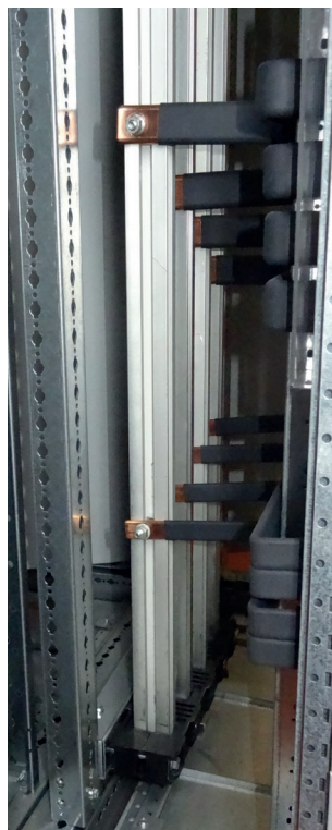
Busbar installed in cable sleeve.
