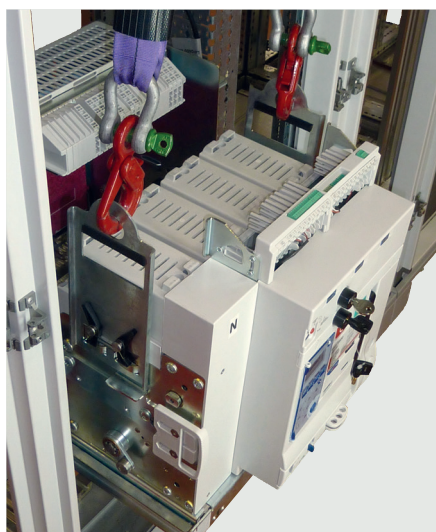
Installing a draw-out DMX 3 in its base.
