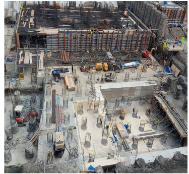
a car park and vital plant equipment, hence a range of Sika products were used to provide the maximum waterproof protection to its reinforced raft slab. These included Sikaproof® A-12, a highly-durable, watertight membrane, and Sika® Watertight Concrete powder, a powerful state-of-the-art admixture. SikaSwell®-A profiles, which swell in contact with water, were used to seal the basement's construction joints.
